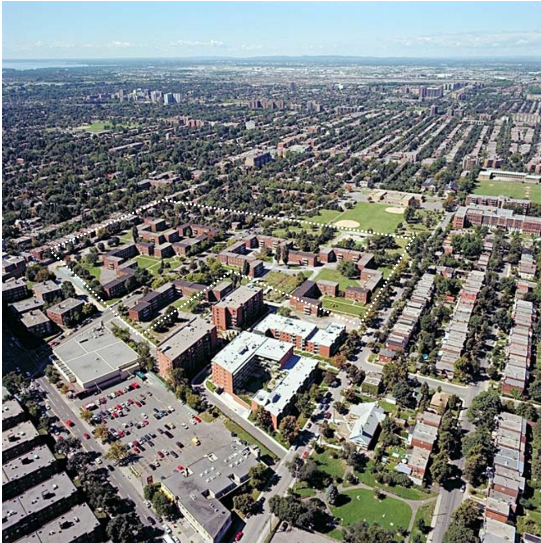
View looking north. The dotted line shows the area slated for redevelopment. (photo Studio Graetz)
