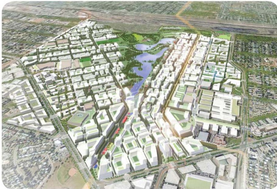
AERIAL VIEW OF BLATCHFORD REDEVELOPMENT [1].
