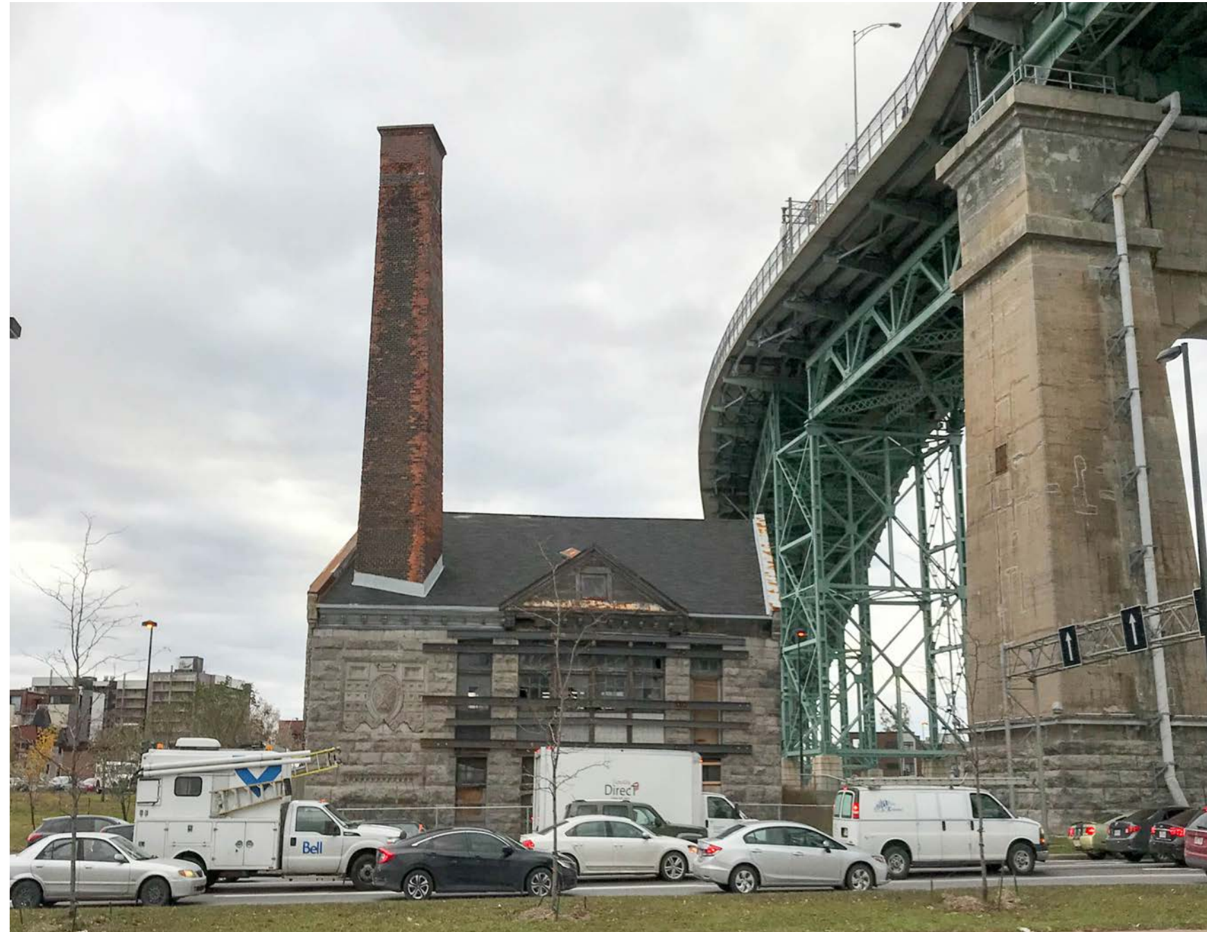
La station de pompage Craig
