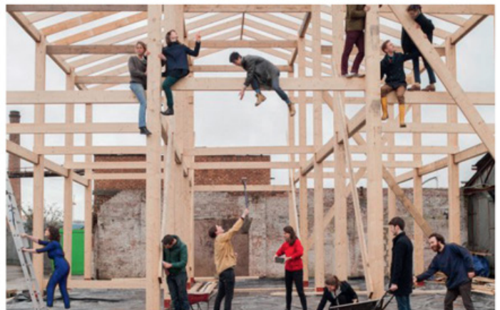
Image of Assemble building the Yardhouse in London courtesy and copyright
