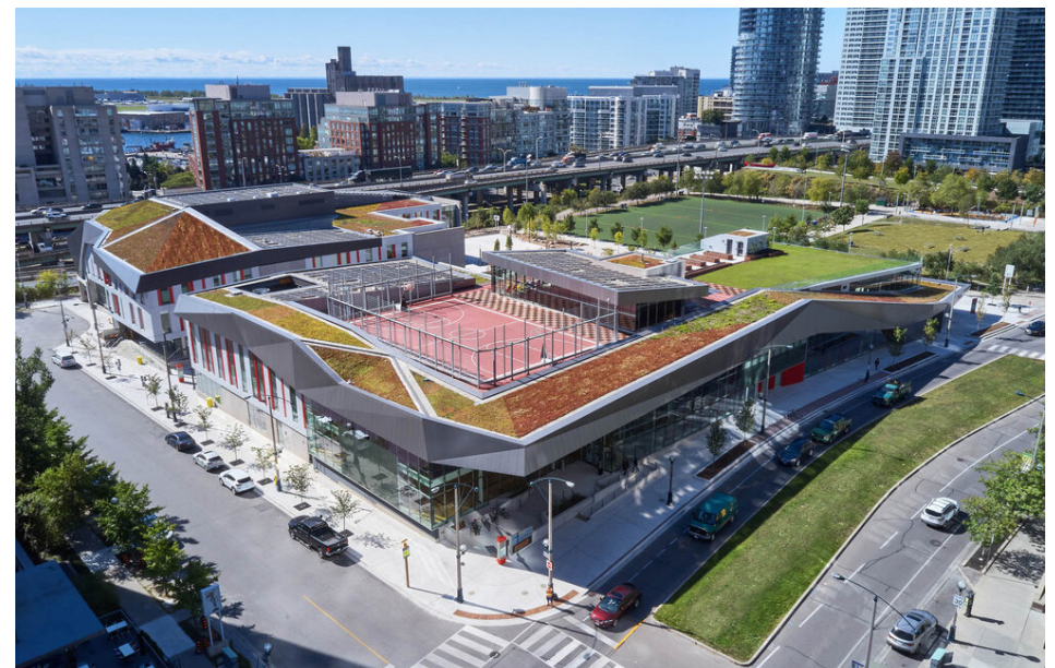
Le Canoe Landing Campus , à Toronto © ZAS Architects
