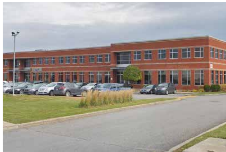
Fig. 72. ADT Security Services et Johnson Controls (Source: Google Street View, 2019)
