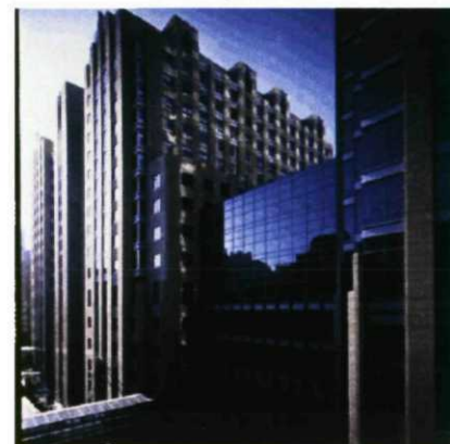
North Western Memorial Hospital
