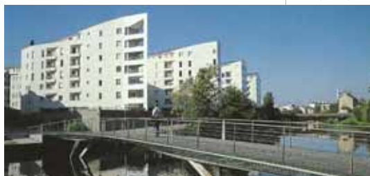
147 | PONCEAU, REINES, FRANCE
