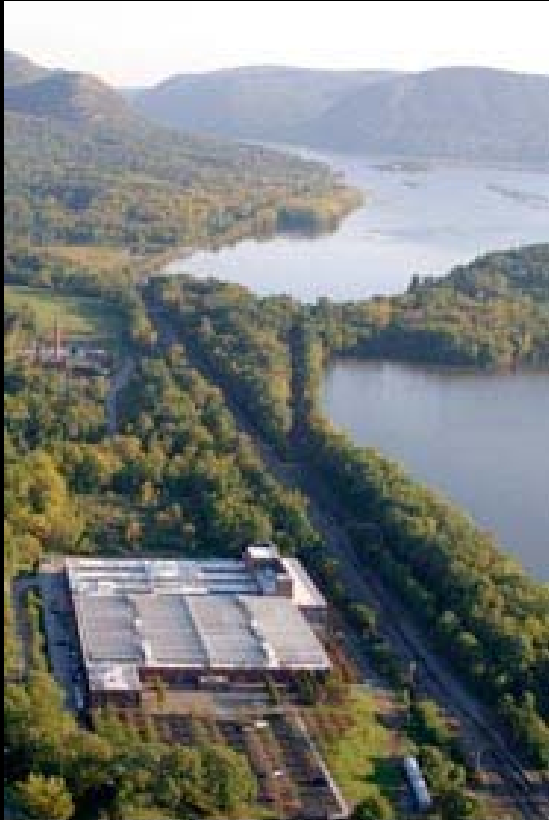
Dia:Beacon, during renovation. Photo: Michael Govan.
