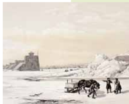
Figure 1.11 Construction du pont Victoria, 1858.
