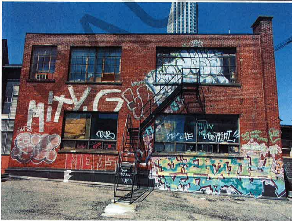
Photograph No. 45: Graffiti art on masonry facade (south façade – roof level)
