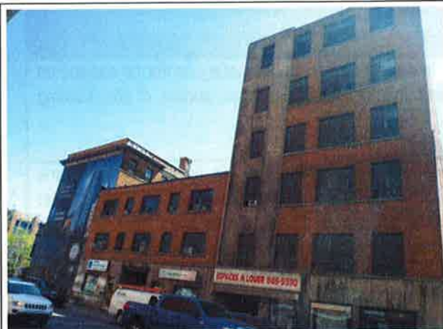
Photograph No. 3: General view of the north façade of the 1162 (far left) and 1180 building
