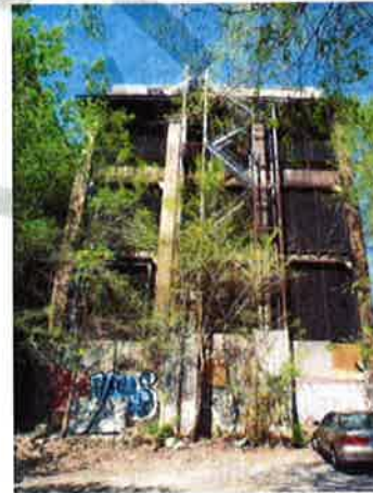
Photograph No. 6: General view of the south façade of the 1162 building
