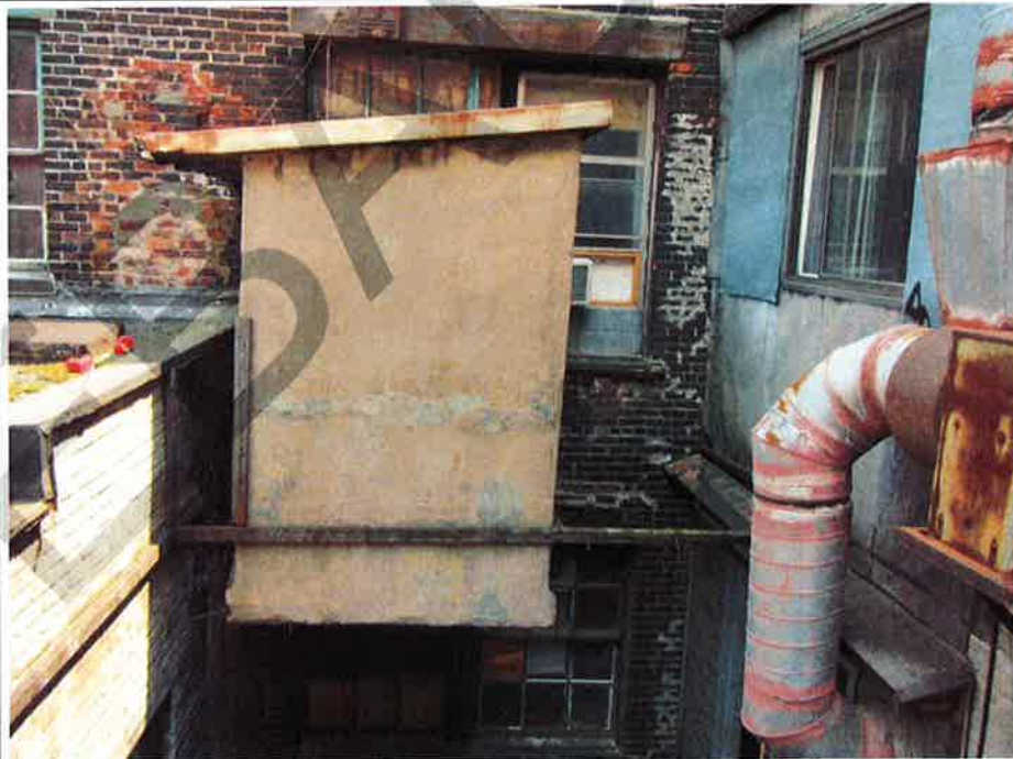
Photograph No. 74 : Building 1180: Overhanging room above courtyard (roof level)
