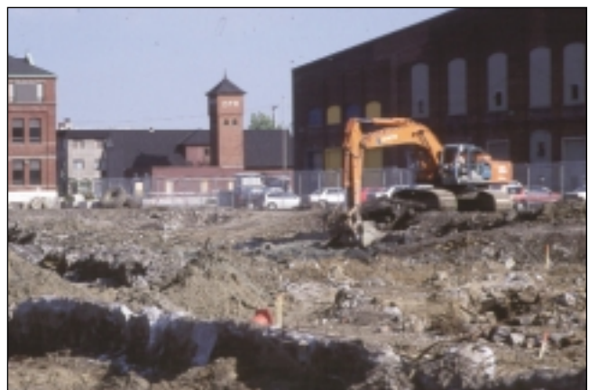
Cleanup at Angus Shops site, 1998
