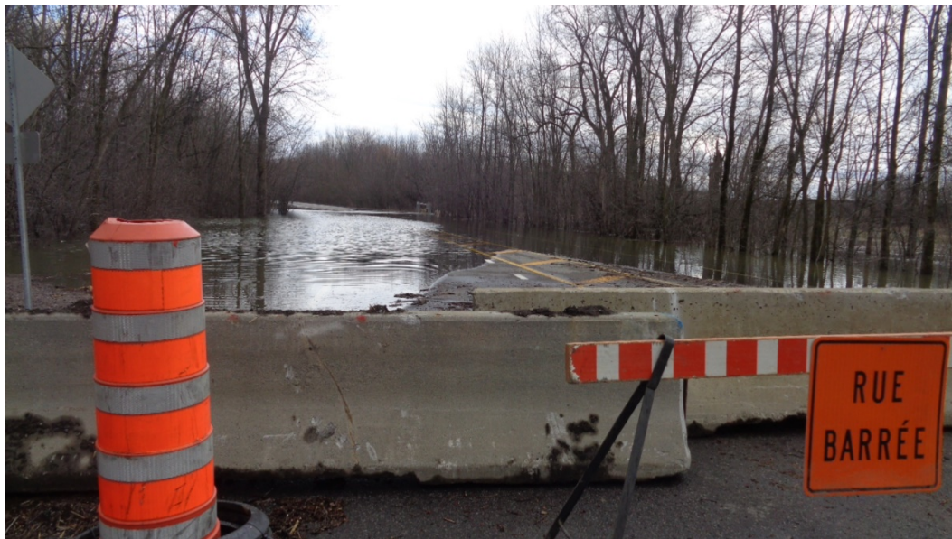
1: As of April 25 th , 2017, the Anse-à-l'Orme Road had been closed for three days due to flooding (above).
