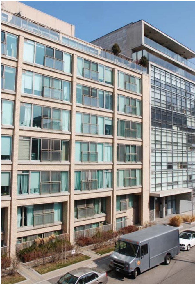
Continuous street wall.
