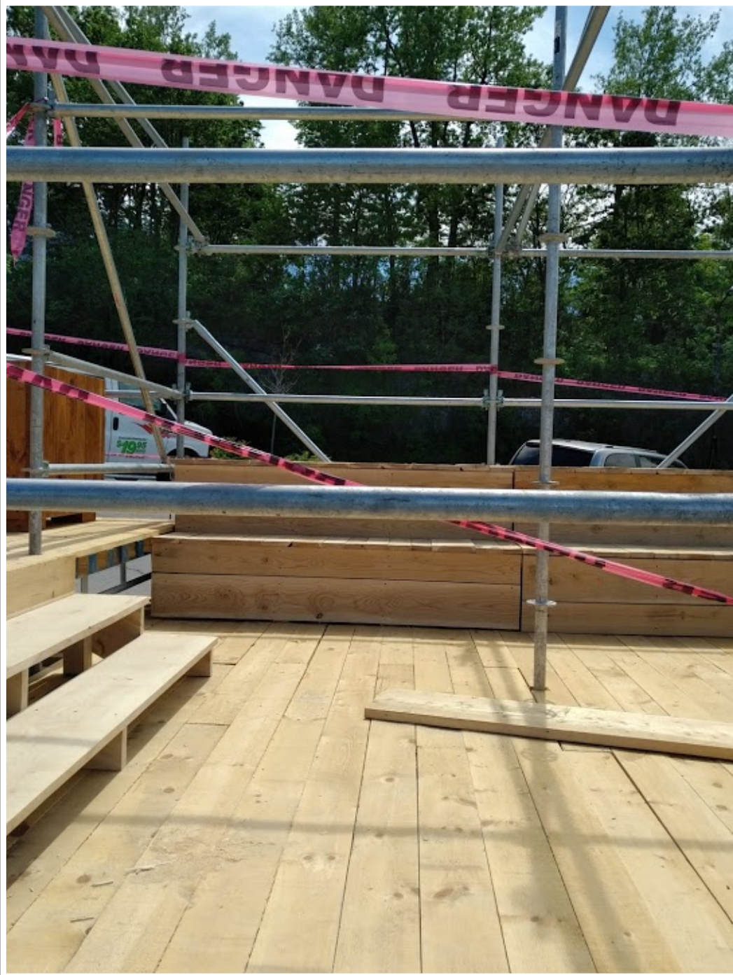
Café Suspendu under construction at C-H Lookout
