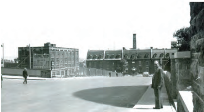
Angle des rues Mansfield et De LaGauchetière, c. 1952, tiré de Anthony Clegg (2008), The Mount Royal Tunnel. Canada's First Subway , Pickering, Railfare DC Books.
